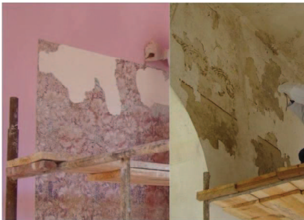
Figure 3: Exploration work on the left side room of the hall (left) and in the hall of the right lateral (right).
